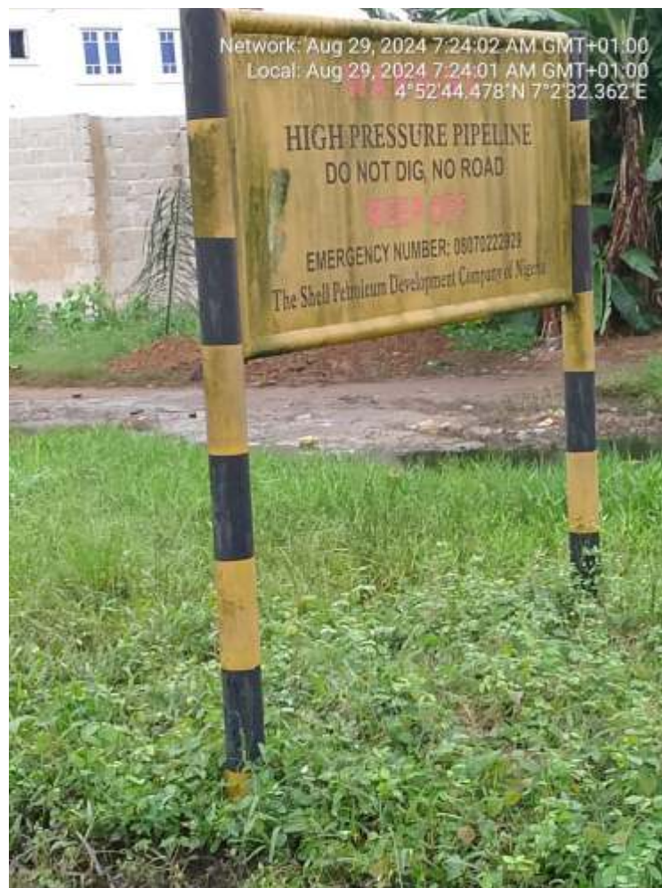
High pressure pipeline near inhabited area
